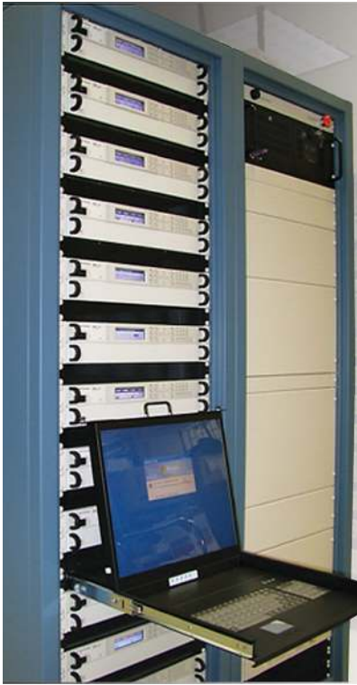
Figure 12. The rack on the left uses 12 Keysight E4360A SAS units to deliver 24 channels of simulation
